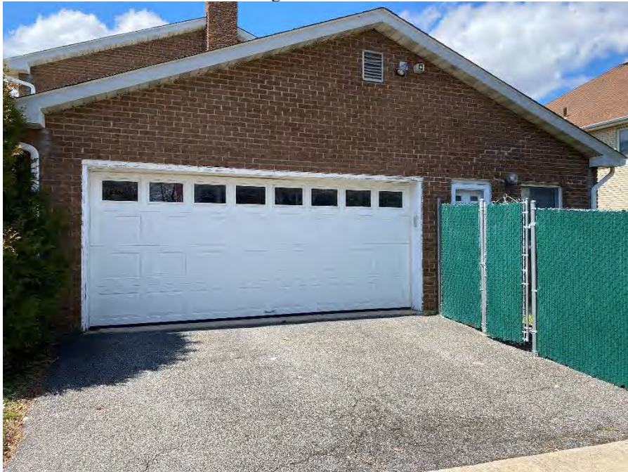
Photo Log #1b – Residence (reported disposal of waste, SEMS-Archive and HSWDS listings). 45 Washington Avenue. High Risk Site No.1: H#1.
