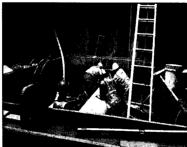
Installation of a 24" Hobas Pipe via Sliplining
