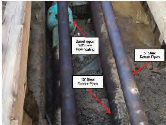
*Figure 1. Excavated Transmission Feeder Pipe.*
