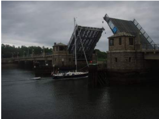
BAYVILLE BRIDGE, BAYVILLE, NY
