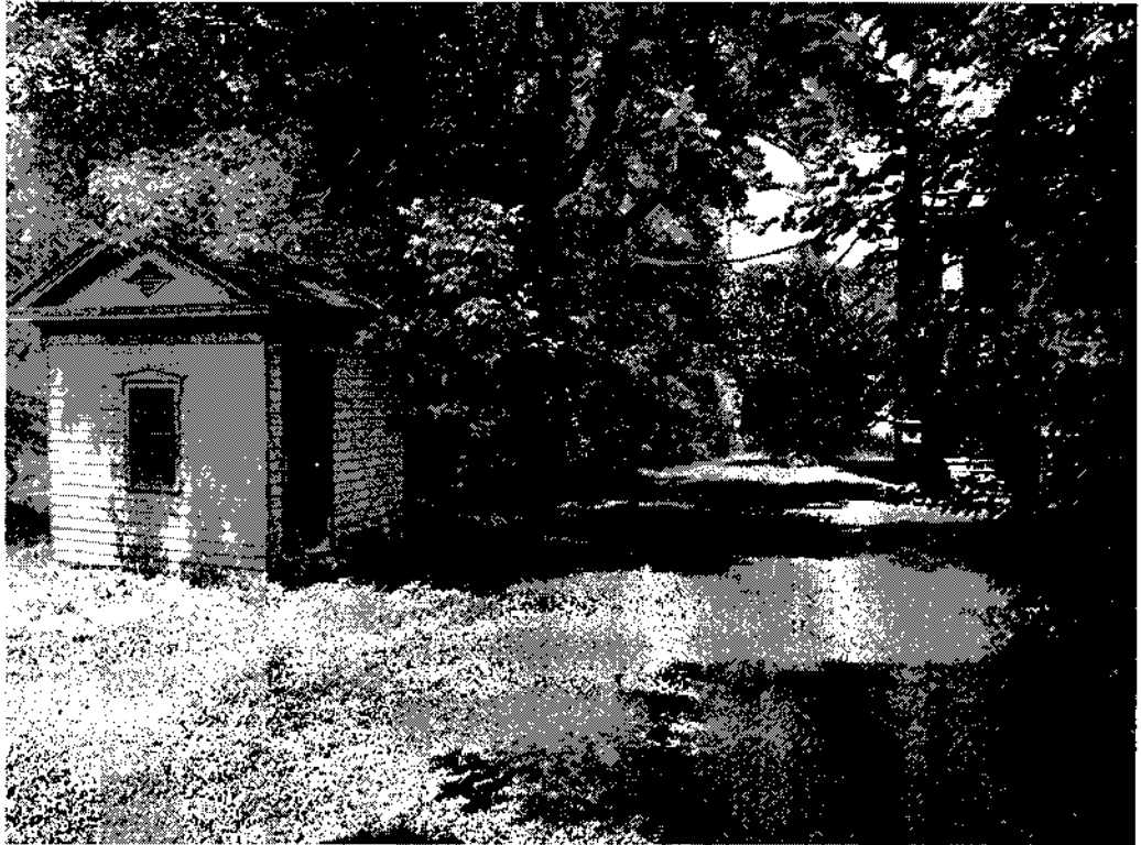
Photo 6. The 1865 Crocheron Privy (left) is a relocated and reconstructed structure on Block 4441a now situated behind the Guyon Store and Tavern (c. 1819/1839). As planned, a proposed sewer line will cross the privy's current site. However, since the building is supported on cinder blocks, it temporarily could be moved out of harm's way or be relocated. (Geismar 8-21-13)
