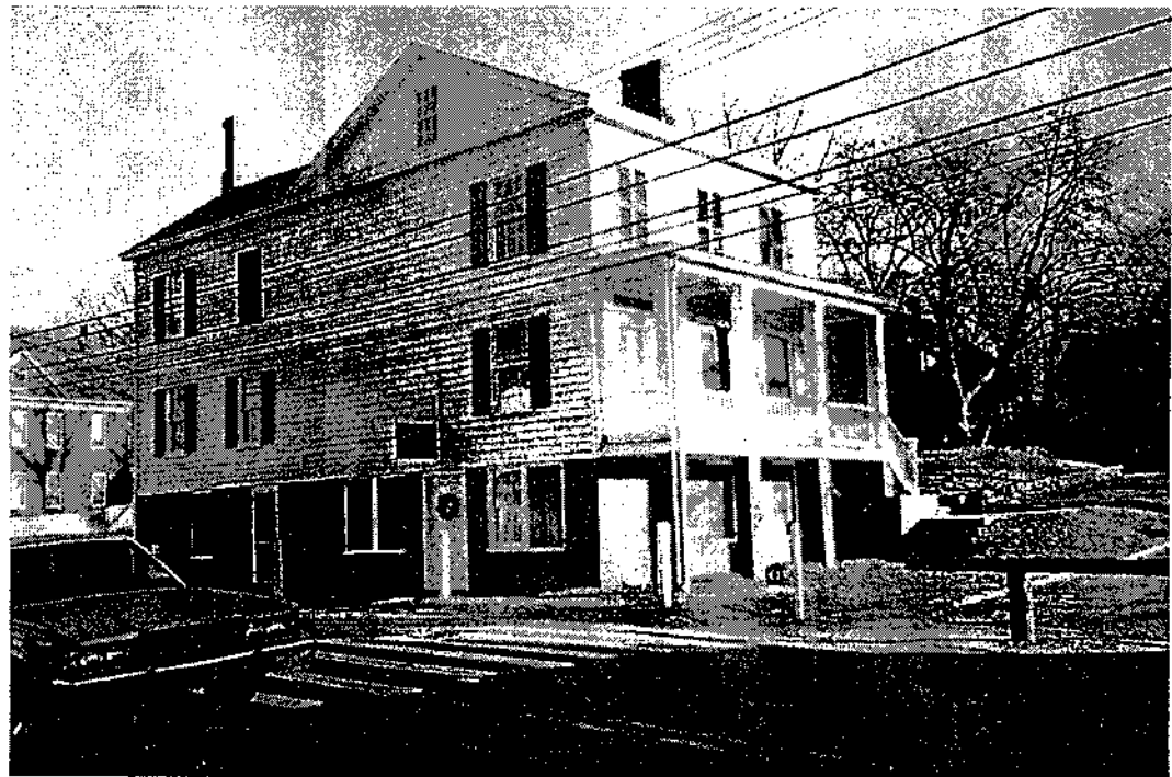
10 The Bennett House from Richmond Road. (Geismar 12/2000)
