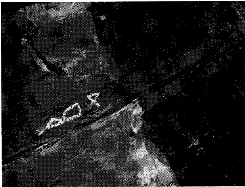
Fig. 10. Strake F, Frame 40 heavily affected by corrosion damage.
