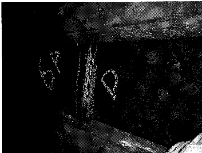
Fig. 7. Heavy corrosion expansion (in chalk) on Strake D at Frame 6.
