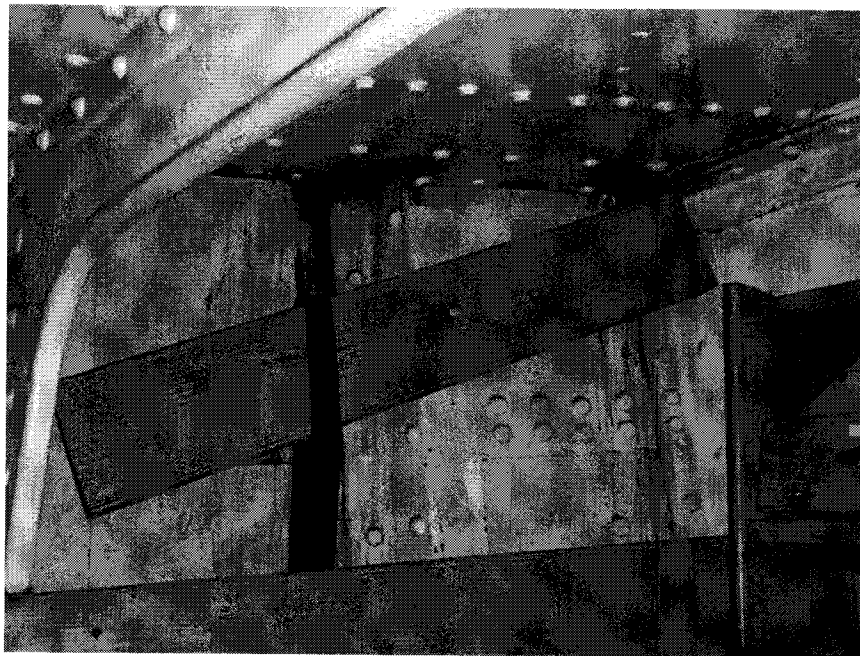
Fig. 62. Collision bulkhead port bounding bar (right side of photograph) to side shell connection.
