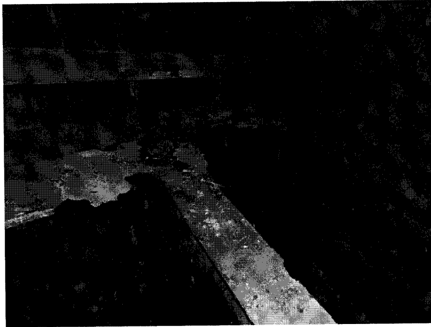
Fig. 45. Starboard panting stringer wasted by corrosion. After panting beam in foreground.
