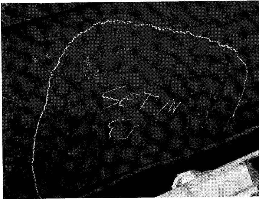
Fig. 70. Strakes F & G set in with plating butt affected. Seam is not open.
