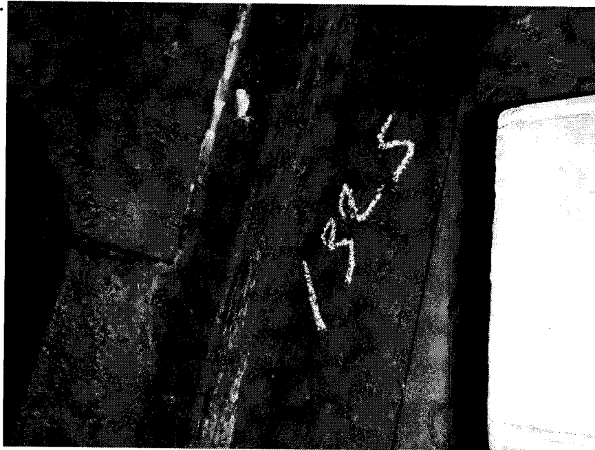
Fig. 46. Heavy corrosion expansion at Frame 132.5.
