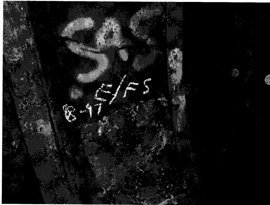
Fig. 33. Seam condition at Strakes E/F, Frames 97-98.
