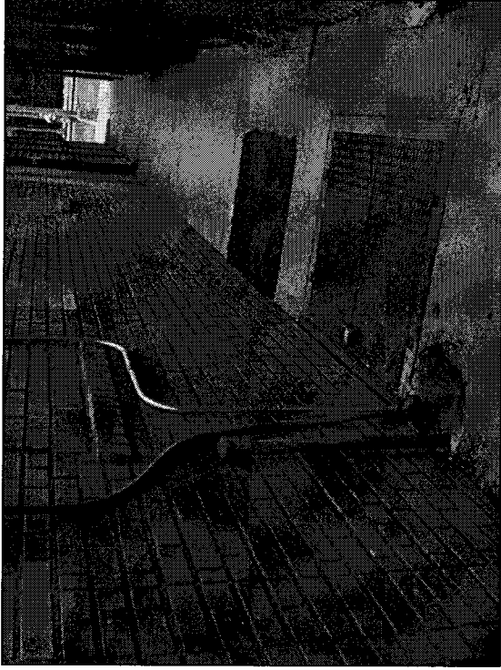
Photograph 2. A vent pipe and fill port for the fuel oil storage tank in the building's basement.
