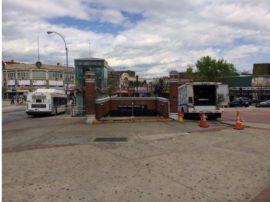
Photo Log #1 – View of the Hunts Point Avenue Train/Subway Station (historically included as gas station), Hunts Point Ave. and Southern Blvd. High Risk Site No: 1.
