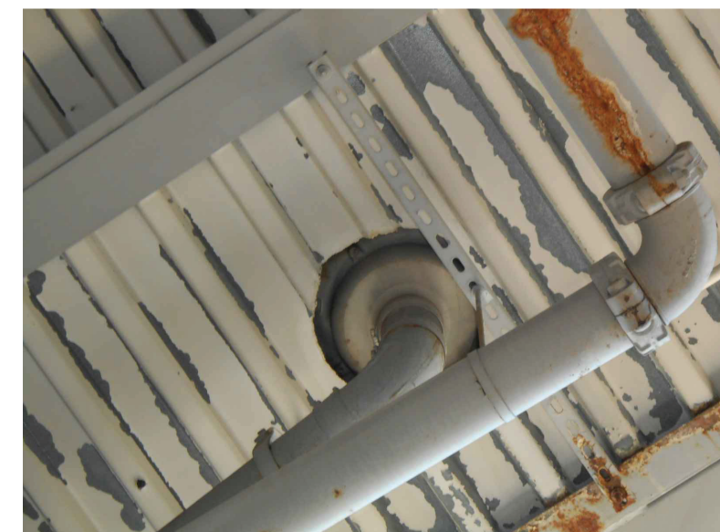
TYPICAL ROOF DRAIN & PIPING
