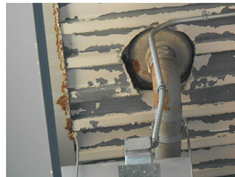
TYPICAL ROOF DRAIN PENETRATION
