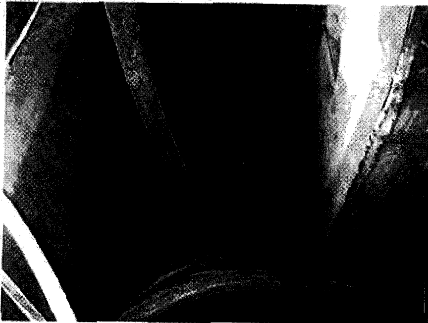
Photograph #6 – View of the bottom of the AST and secondary containment basin. Note thick dark staining.
