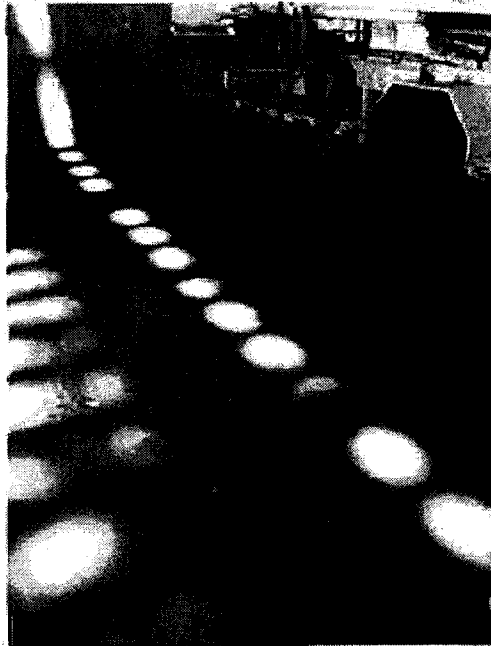
Photograph #12 – View of typical staining found at the site.
