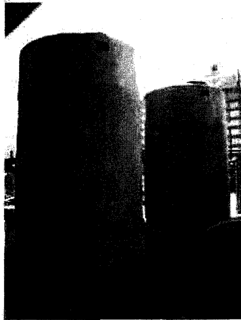
Photograph #4 – View of two (2) 6,250-gallon plastic potassium acetate solution ASTs.
