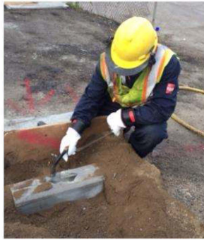
Break out window on each top duct found. Strike Away From the center.
