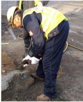
Find edges & visualize all ducts. Remember that There could be several across and underneath. Keep area clean, so you can tell configuration.
