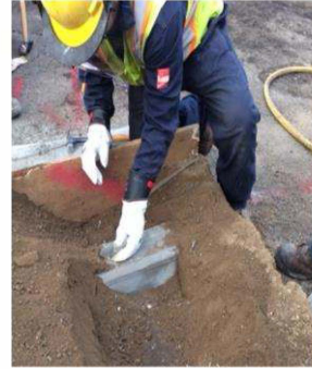
Insert Micarta "half moon" protective insert in windows on ducts. Continue breaking top rows of ducts in a horizontal direction sliding Protective Micarta down the run while breaking the top & sides.
