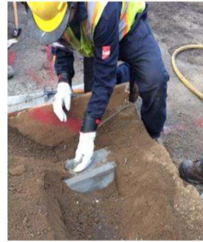
Insert Micarta "half moon" protective insert in windows on ducts. Continue breaking top rows of ducts in a horizontal direction sliding Protective Micarta down the run while breaking the top & sides.
