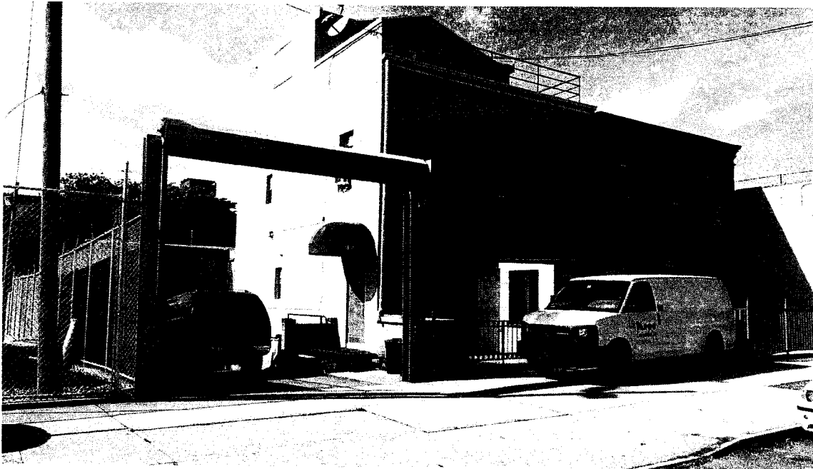
#12 – Vardo Construction Corp. / 1850 Steinway Street. View from Steinway St. facing west. (Moderate Risk Site No. 6)
