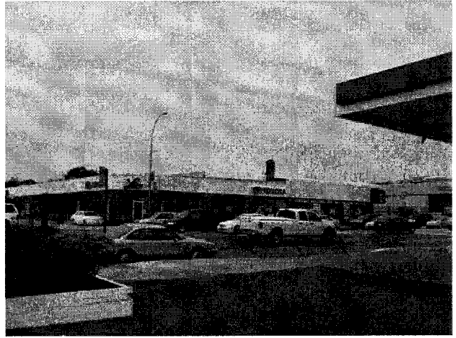
Photo No. 32 – View of Moderate Risk Site No. 30, Lee's Motors Inc., 139-65 Queens Boulevard, Map ID 114.
