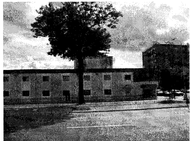
Photo No. 36 – View of Moderate Risk Site No. 34, 13904 Queens Boulevard, Map ID N/A.
