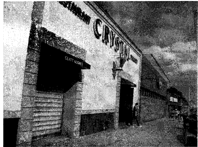
Photo No. 38 – View of Moderate Risk Site No. 36, 13831-13833 Queens Boulevard, Map ID N/A.
