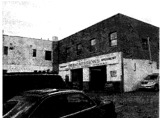
Photo No. 40 – View of Moderate Risk Site No. 38, 144-01 Hillside Avenue, Map ID N/A.
