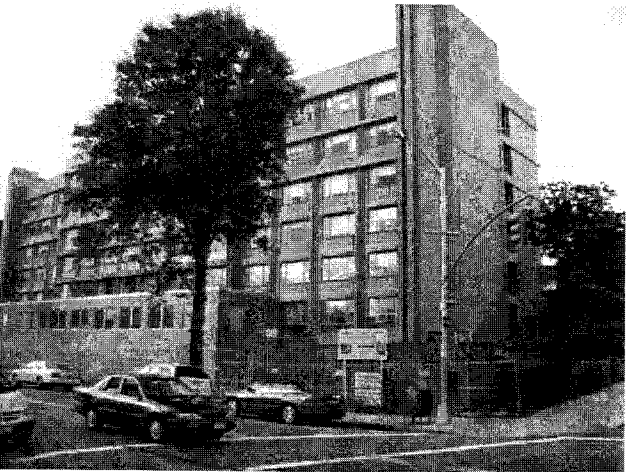
Photo No. 5 – View of Moderate Risk Site No. 3, Margaret Tietz Center for Nursing Care, 164-11 Chapin Parkway, Map ID 13.
