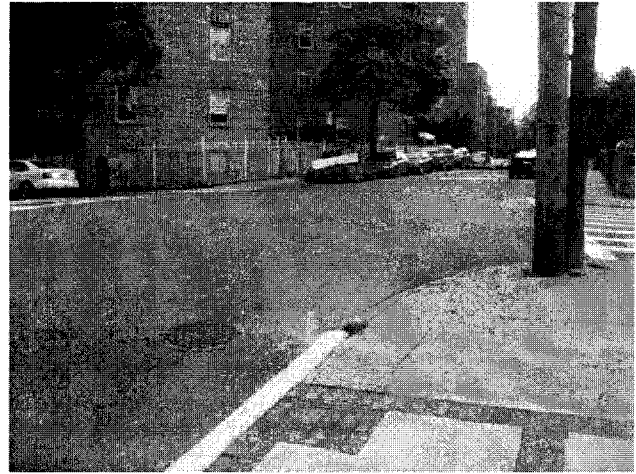
Photo No. 14 – View of Moderate Risk Site No. 12, Manhole 10025, 143rd Street and 85th Drive, Map ID 57.
