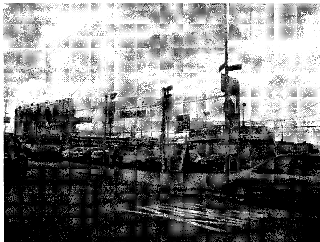
Photo No. 35 – View of Moderate Risk Site No. 33, 138-10 Hillside Avenue, Map ID 121.
