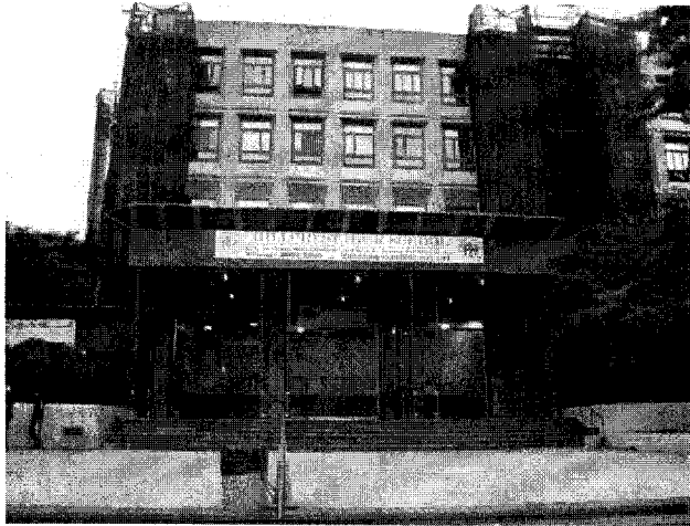
Photo No. 19 – View of Moderate Risk Site No. 17, NYC BD of ED - Hillcrest High School / NYC BD of ED - PS 86Q, 160-05 Highland Avenue / 87-41 Parsons Boulevard, Map IDs 60 and 70.
