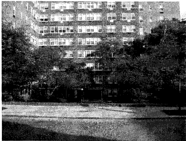
Photo No. 9 – View of Moderate Risk Site No. 7, Commercial Building, 164-20 Highland Avenue, Map ID 41 (Currently residential).
