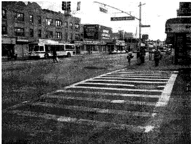
Photo No. 23 – View of Moderate Risk Site No. 21, Manhole TM908, Parsons Boulevard and Hillside Avenue, Map ID 84.
