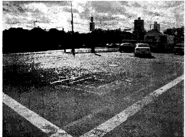
Photo No. 16 – View of Moderate Risk Site No. 14, Manhole #1360, Queens Boulevard and 84th Drive, Map ID 58.
