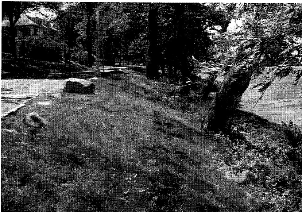
Photo 17. Location of Outfall No. 7 at the foot of Hollywood Avenue. View is toward the south, with Shore Road at the left (east).
