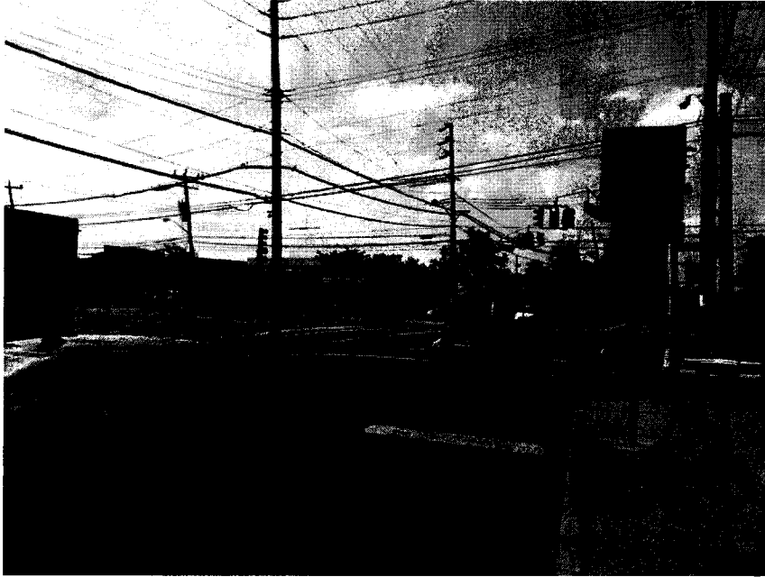
Photo Log No. 13 – CSX Transportation, Inc., South & Forest Avenue, Staten Island, NY (Moderate Risk Site No. 8).
